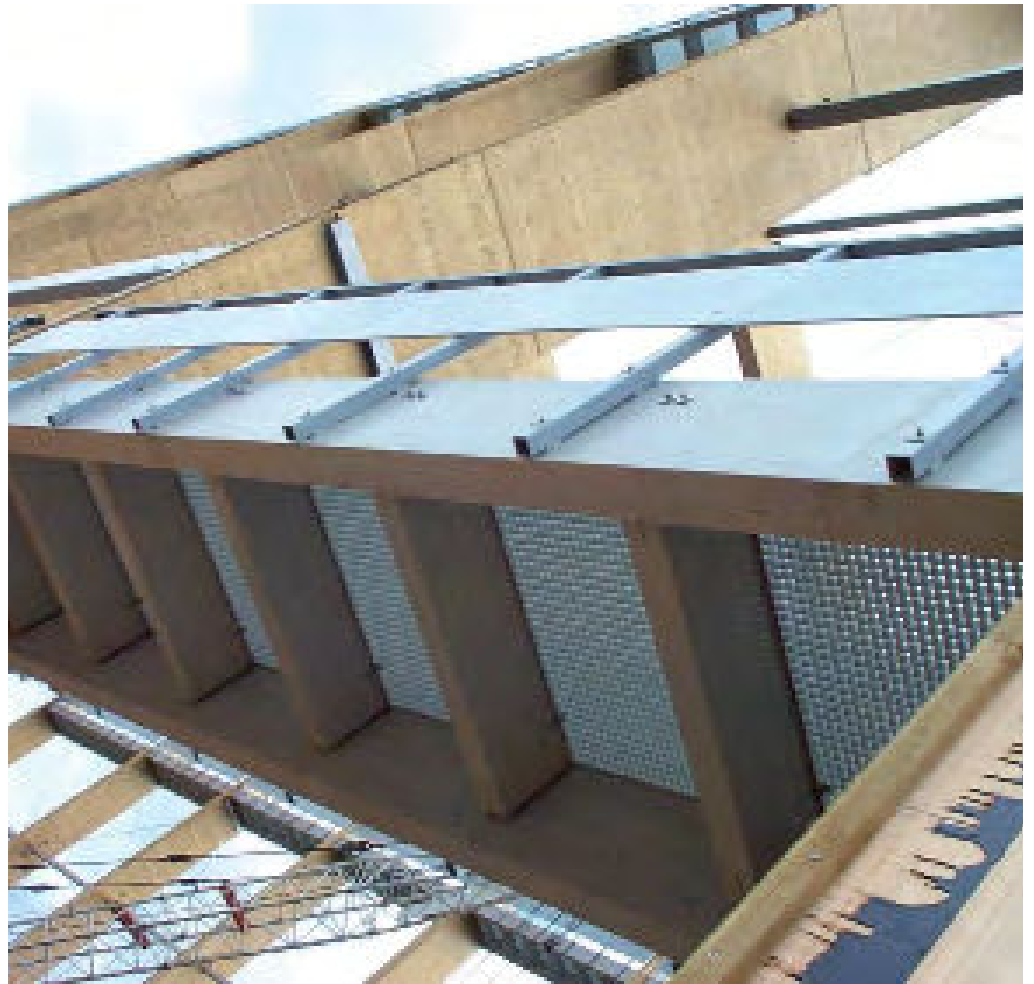
Top: Anti-magnetic field: simply composed of wood and GRP
