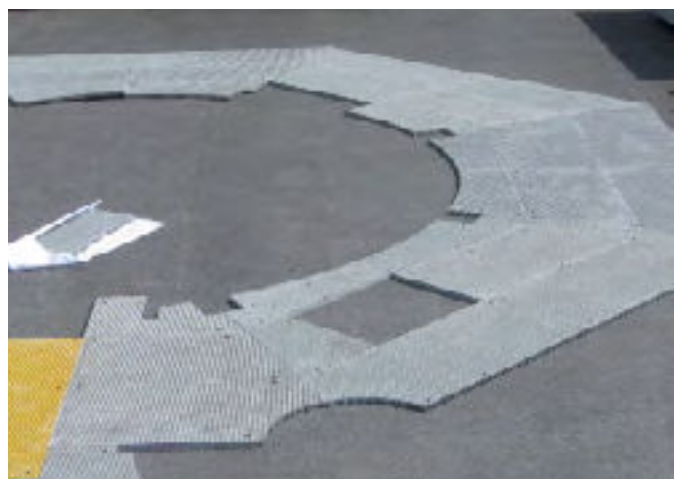
Bottom right: Quality control of GRP grating
